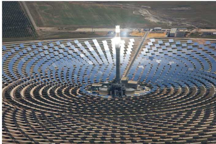
Figure 1-2 Aerial view of Gemasolar power plant [5]
